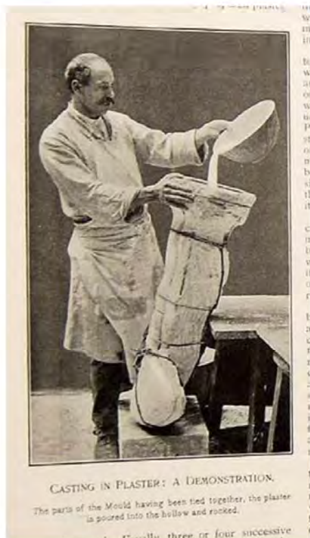
CASTING IN PLASTER: A DEMONSTRATION.—DRAINING THE SUPERFLUOUS PLASTER.
